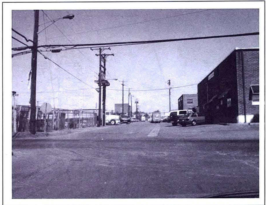
An older industrial area in the Planning Area with parking and loading areas spilling into the street.
