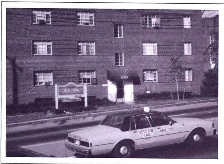
Landscape and facade improvements made to an apartment building.
