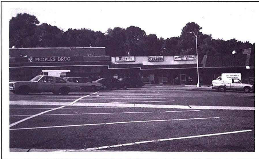
Uncoordinated store facades (also note lack of parking lot landscaping).
