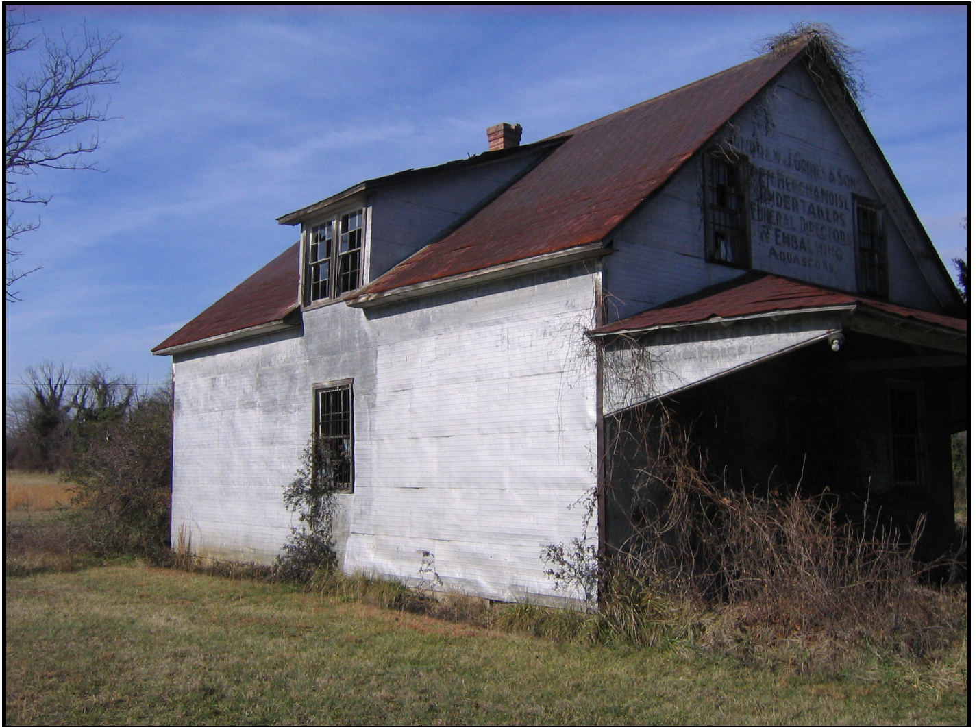
Photo: James A. Cochran Store, c. 1850, view of the south (side) elevation, looking northwest. (January 2008)
