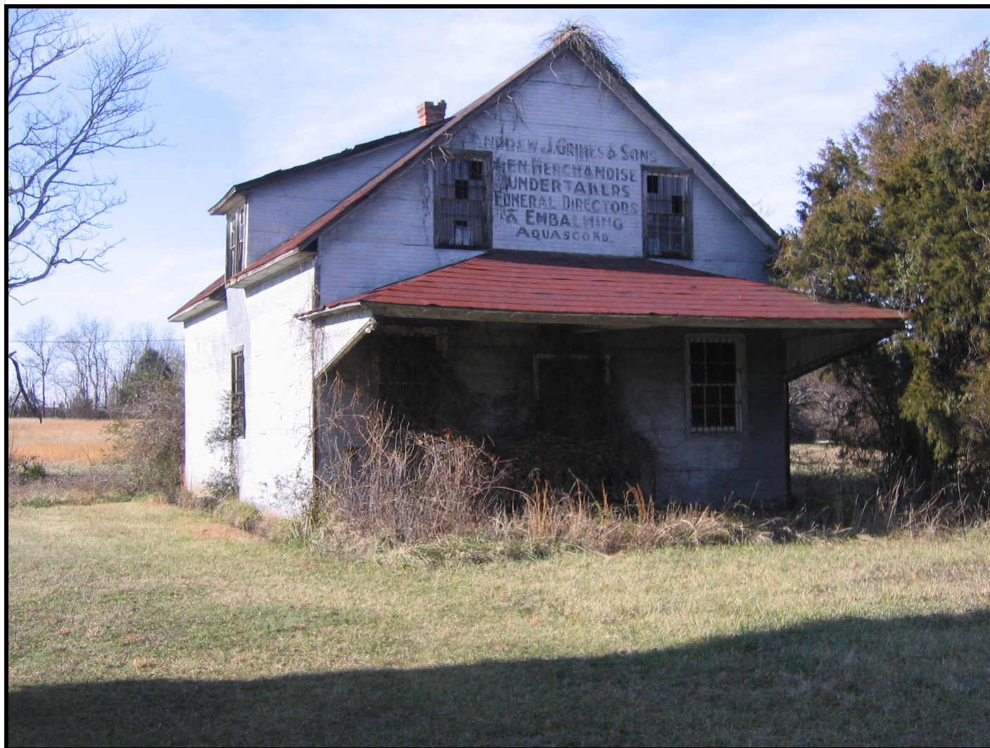
Photo: James A. Cochran Store, c. 1850, view of the façade (east elevation), looking west. (January 2008)
