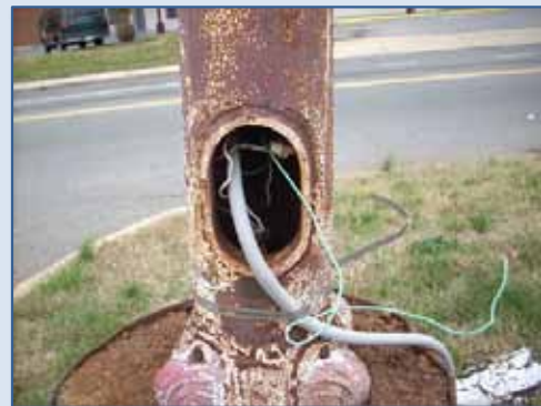
Improper electrical wiring on parking lot lamppost
