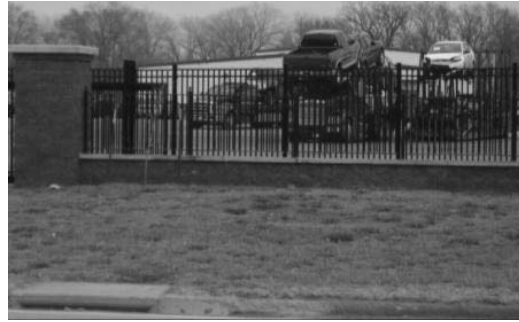
Figure 5. Masonry and wrought iron fencing at auto auction (Kansas City, KS)
