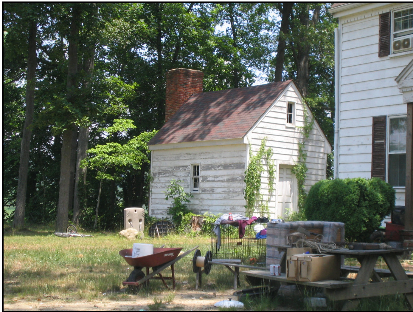
Photo: Outbuilding, southwest corner, looking northeast.
