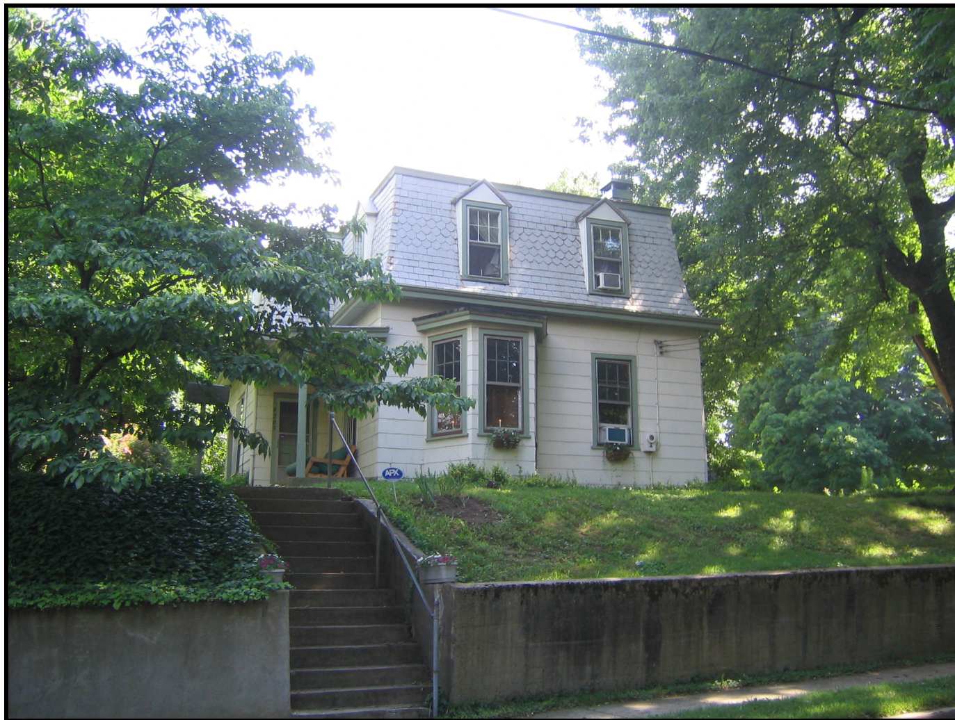
Photo: Rural Cottage at The Highlands, façade (north elevation), looking south.
