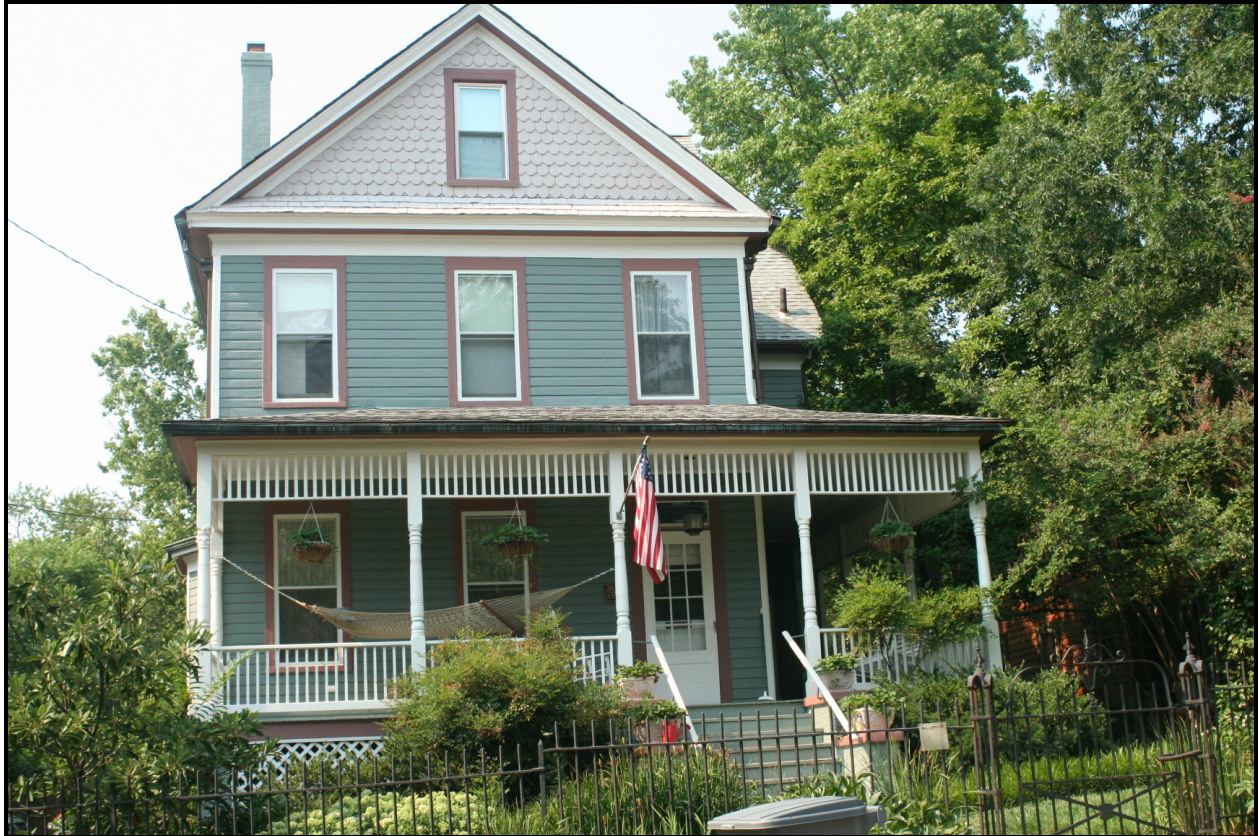
South elevation, Wheelock House (PG: 68-010-31), 4100 Crittenden Street ( EHT Traceries , 2007)
