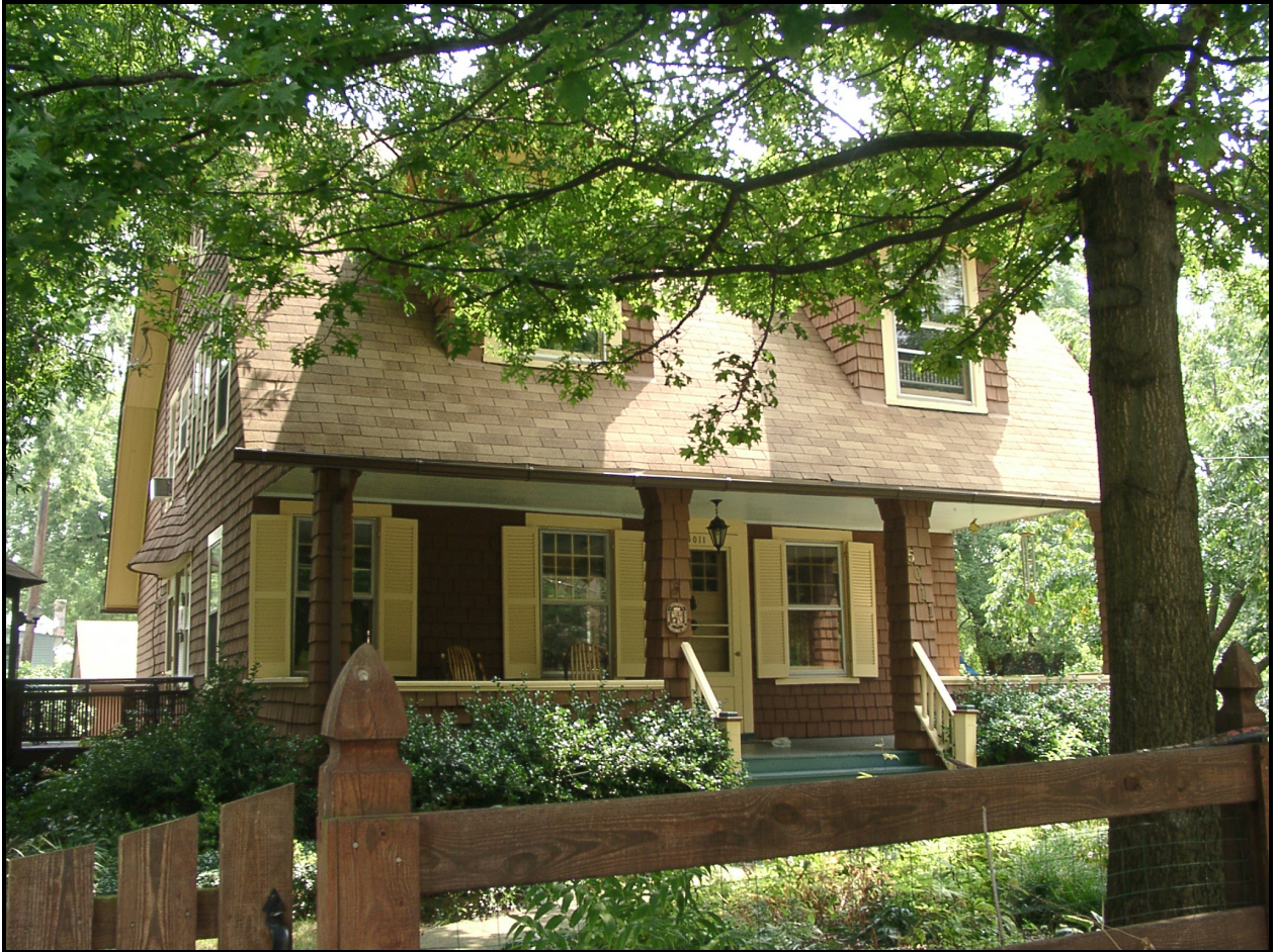
Looking east, Fox's Barn (PG: 68-010-74), 5011 42nd Avenue ( EHT Traceries , 2007)
