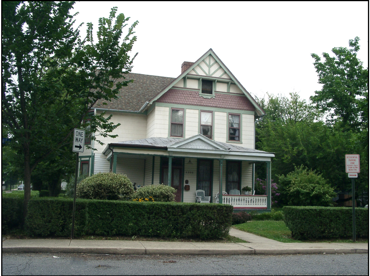
Looking northeast, Welsh House (PG: 68-010-01), 4200 Farragut Street ( EHT Traceries , 2007)
