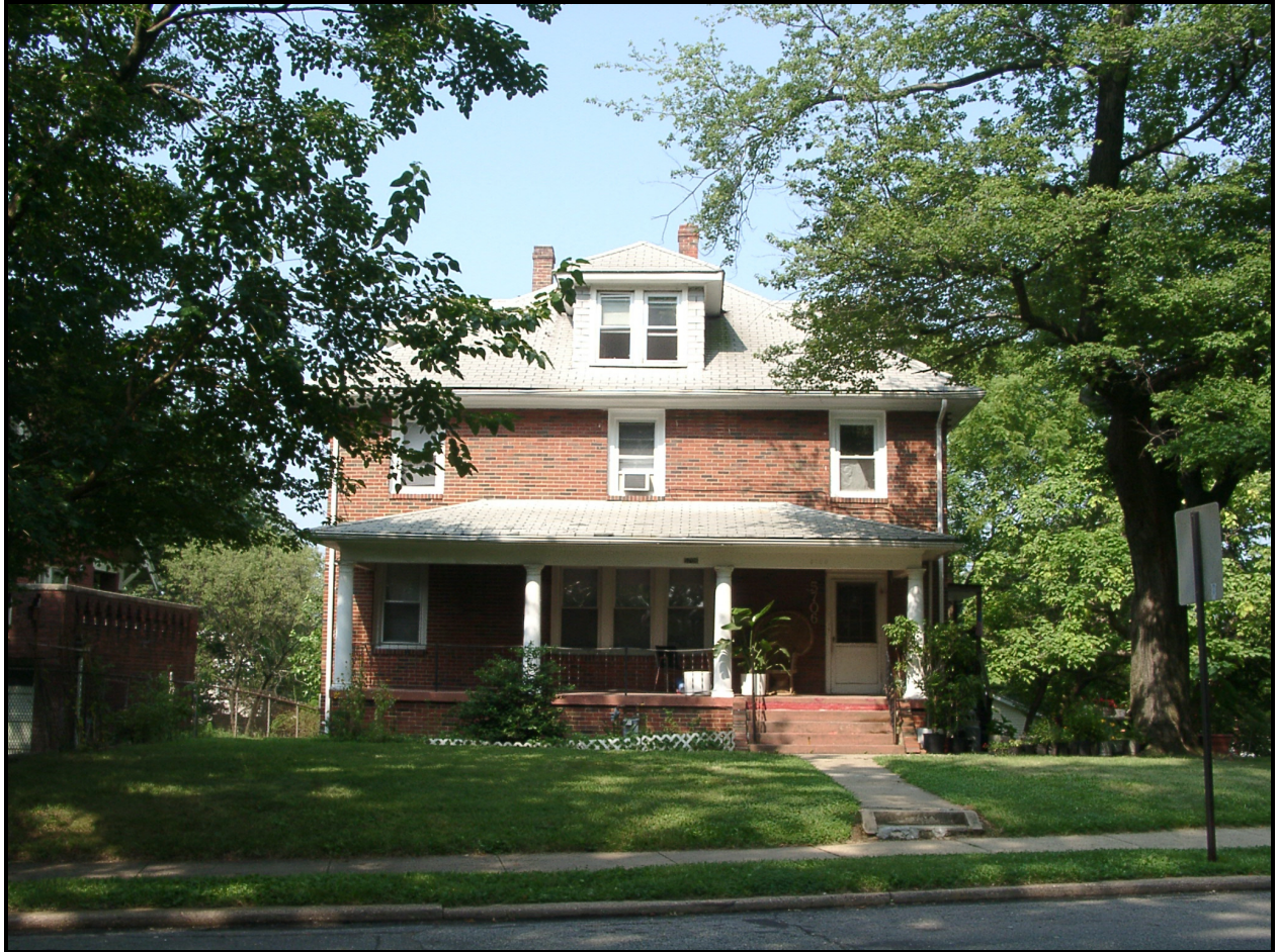
Looking west, 5706 42nd Avenue ( EHT Traceries , 2007)
