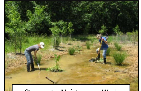
Stormwater Maintenance Work
